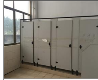
Photo of the sanitary facilities toilet.JPG
