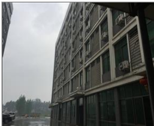
External photo(s) of the production unit(s) office and canteen building.JPG
